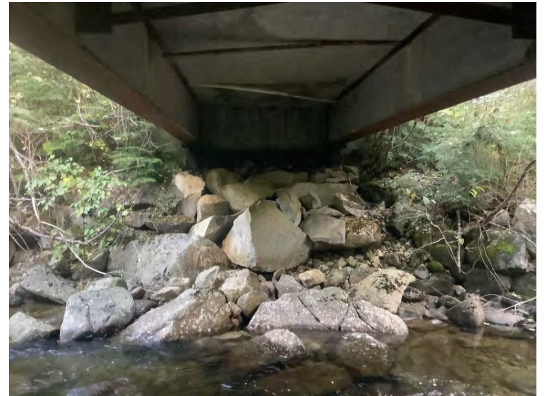
Left Bank Abutment when facing downstream
