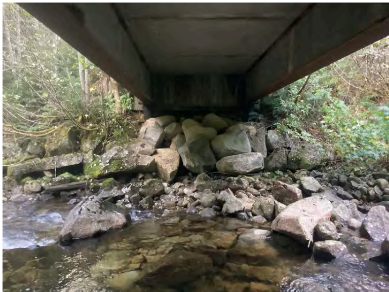
Right Bank Abutment when facing downstream
