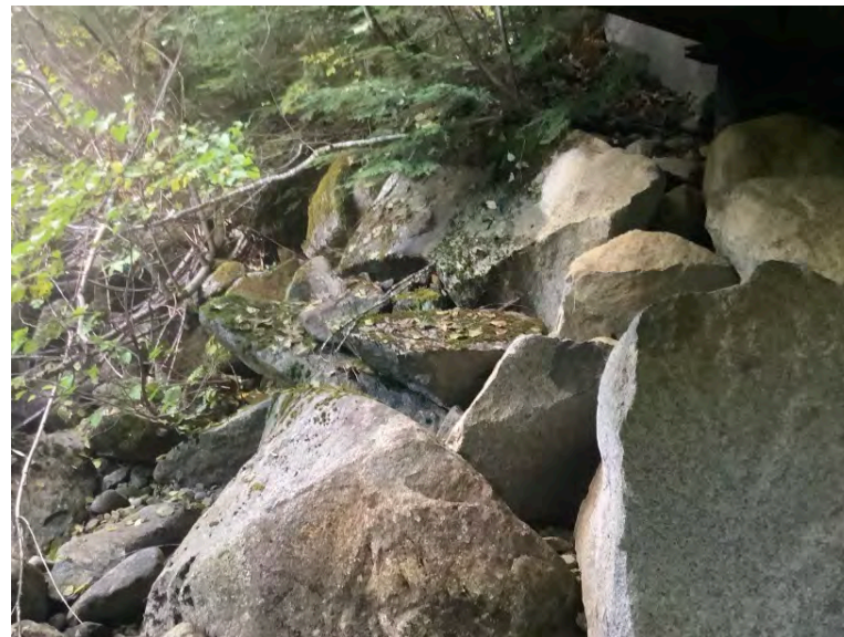
Left Bank Abutment when facing downstream
